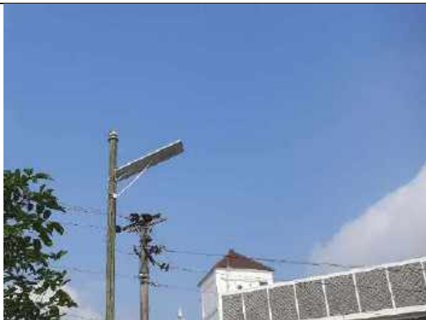
Figure 8. Solar Power for Street Lighting
