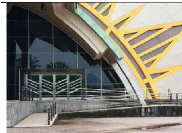
Figure 3. Wheel Chair Access at Sportorium Building
