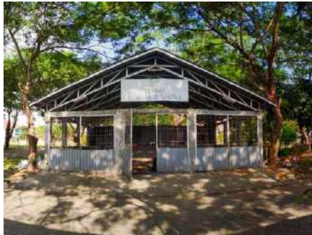
Figure 3. The wastes collection point inside UMY
