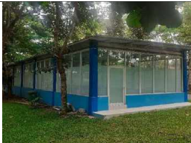
Figure 4. Sewage treatment plant (STP) owned by Universitas Muhammadiyah Yogyakarta
