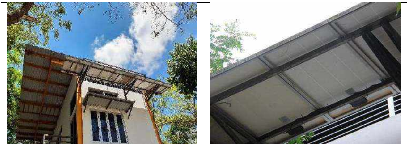
Figure 1. 1 KW PV Monocrystalline Solar Cell in Universitas Muhammadiyah Yogyakarta
