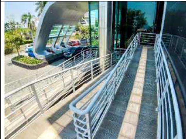
Figure 7. The pedestrian path to the auditorium for disabled people
