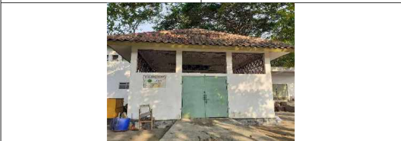
Figure 6. Bioenergy Facility Used to Turn Organic Waste Into Fuel in Universitas Muhammadiyah Yogyakarta
