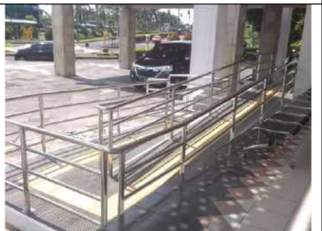
Figure 4. Wheel Chair Access at Rectorate Building
