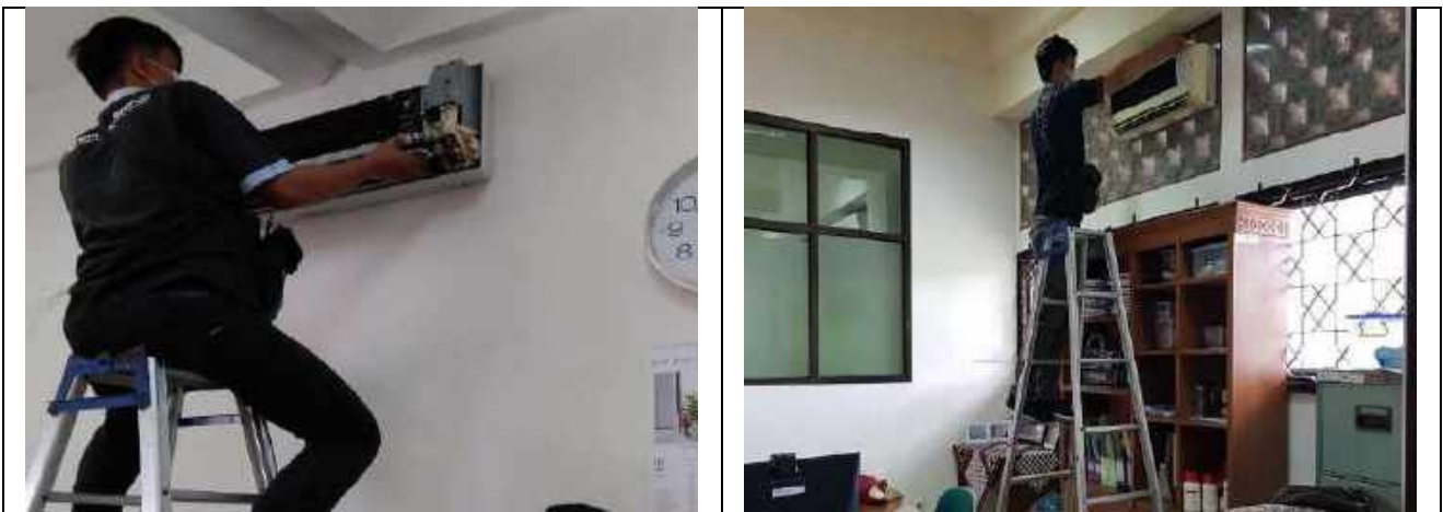
Figure 1. Air Conditioning Maintenance
